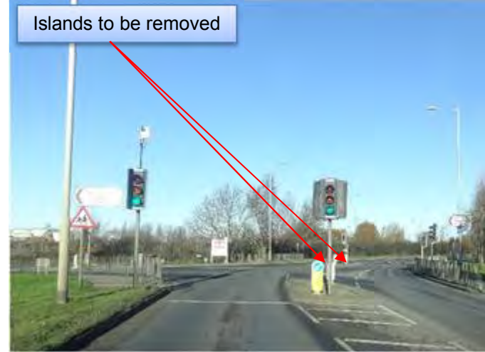
8.4.6.3. – View on junction
