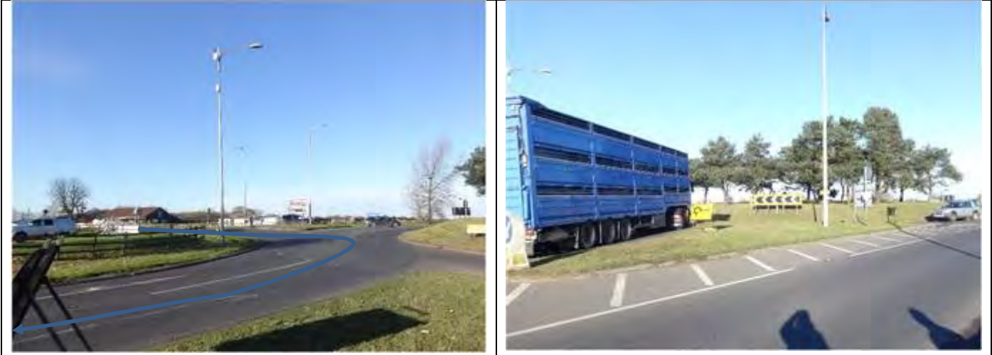
8.6.1.3. – View on roundabout 8.6.1.4. – View on junction
