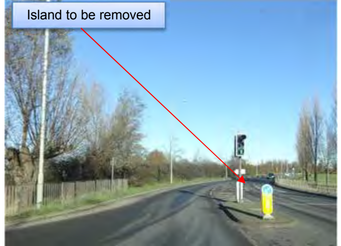
8.4.6.4. – View on junction
