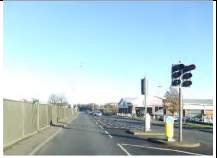
8.4.5.4. – View on junction
